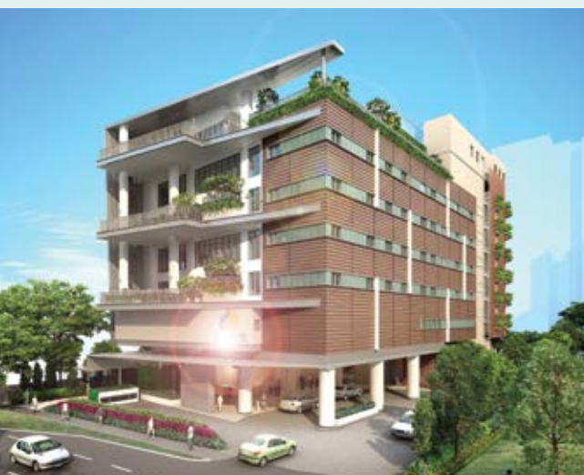
The seven-storey Pioneer Polyclinic will be a future-ready centre designed to be a health-promoting classroom with an open rooftop and communal spaces for community engagement.
