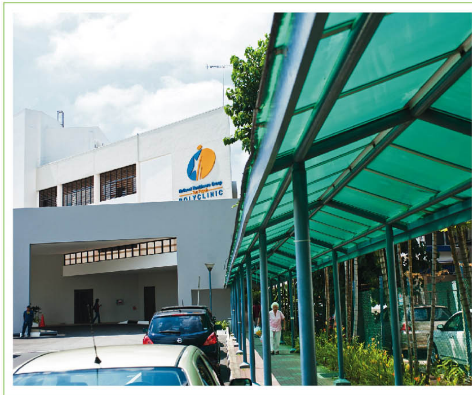
The newly upgraded Toa Payoh Polyclinic.
