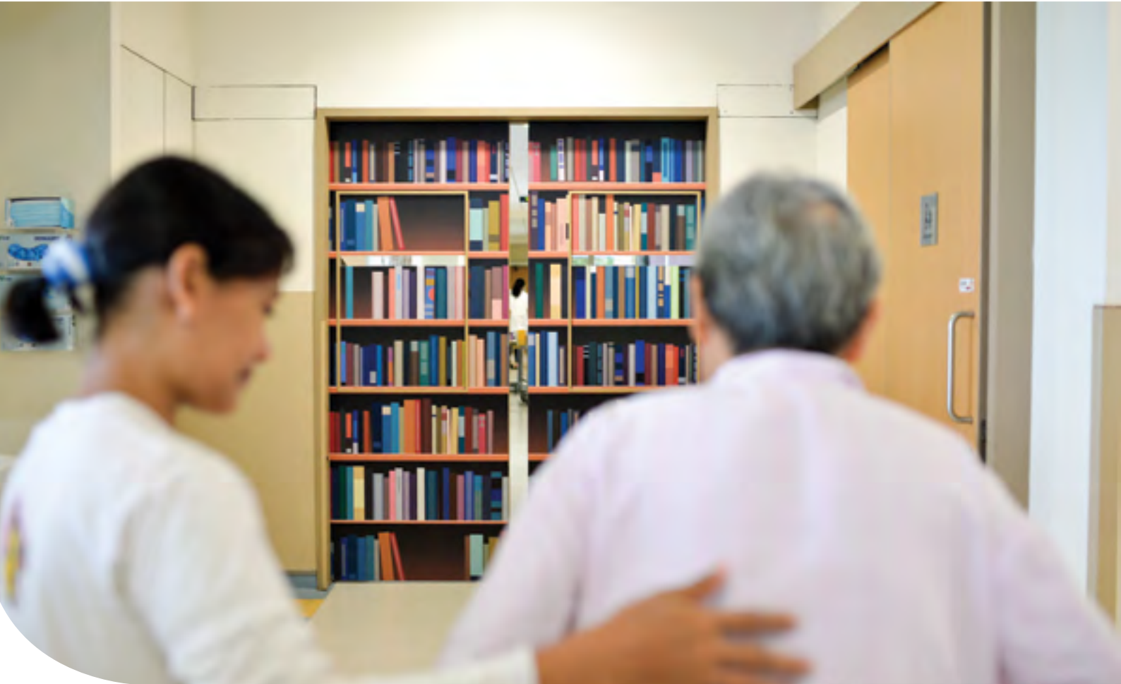
Doors at Khoo Teck Puat Hospital's dementia ward, such as the one above, are painted to look like bookshelves so that patients won't be tempted to walk out or become angry when they are not allowed to. Source: The Straits Times © Singapore Press Holdings Limited. Reproduced with permission.
